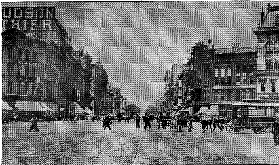
STREET VIEW, LOOKING NORTH ON WOODWARD AVENUE, FROM CAMPUS MARTIUS.
